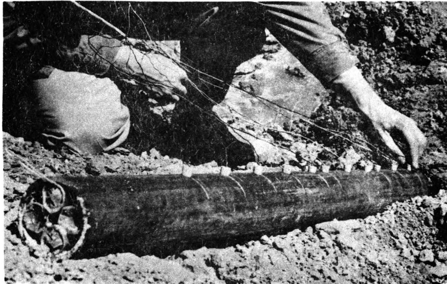
Charge container with cork pins and dynamite primer.
